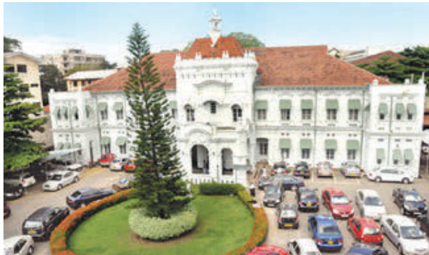
Vintage NHSL Building
