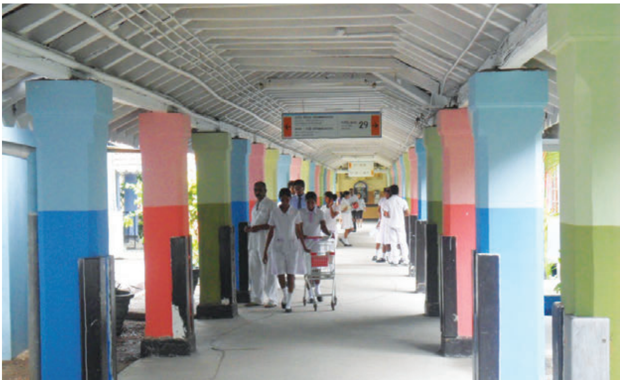
Painting Adjacent Corridors
