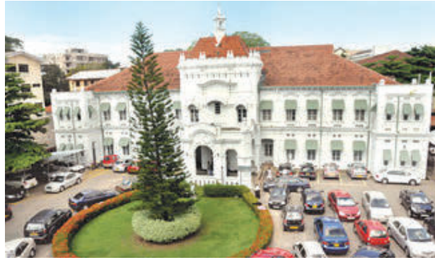
Vintage NHSL Building
