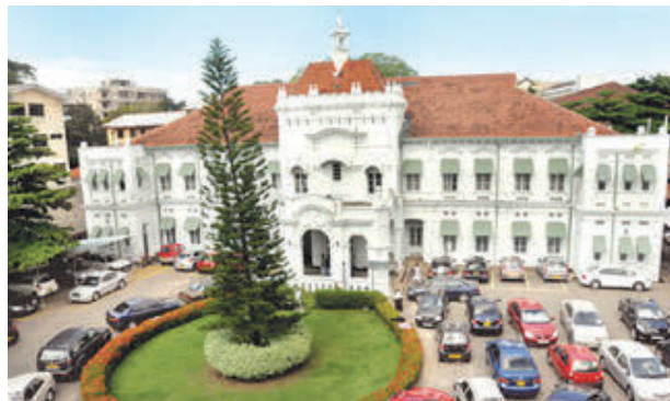
Vintage NHSL Building
