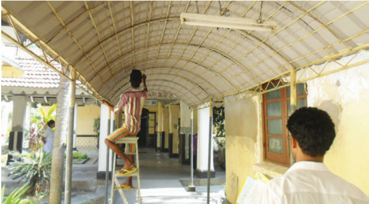
Painting the Columns
