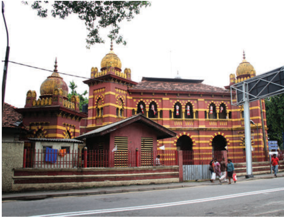
Victoria Memorial Building - 1903
